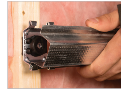
Engage furring channel into either claw, then squeeze channel to engage the claw
